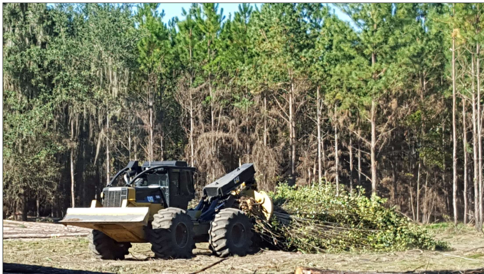
Separating the biomass from the pulpwood and chipping on site
